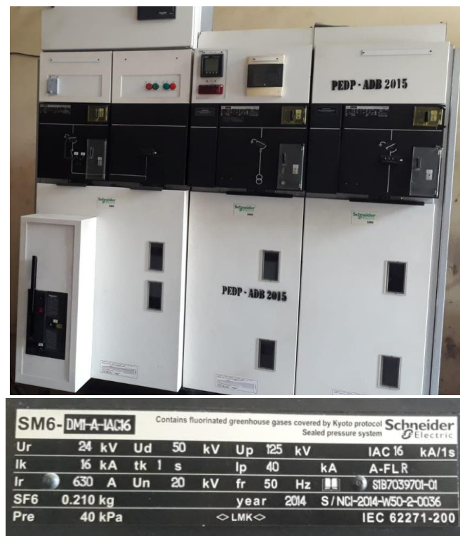
Figure 3. 24 kV CB SF6 630 Amp Cubicle Model
