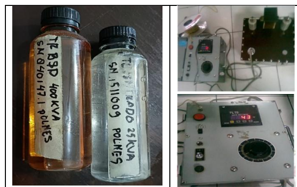
Figure 6. Transformer Oil Sampling Data and Breakdown Voltage Test on Distribution Transformer 25 kVA Phase 50 Hz 400 V/ 20 kV - TR. Centrado 25 kVA SN. 1511009
