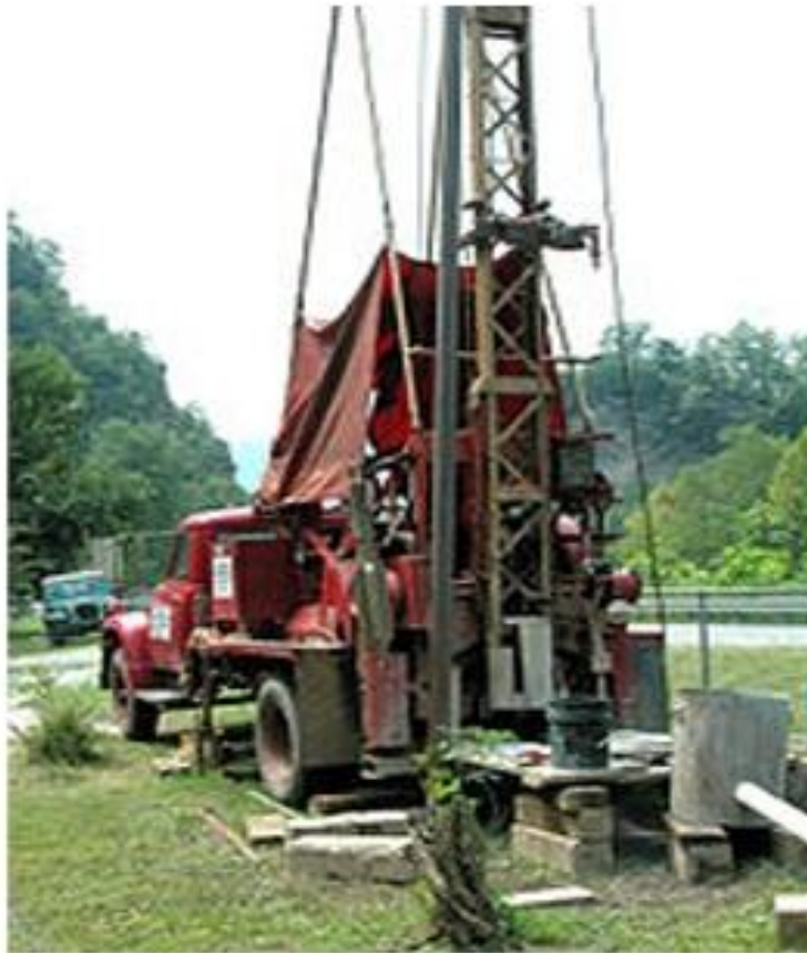
Fig. 3 A drilled well under construction.
