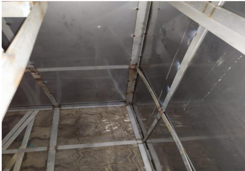
Figure 2. The bottom frame of the rainwater storage box with a flat position and double frame, a foothold for the barrier like a brick, as a barrier so that the container does not quickly sink
