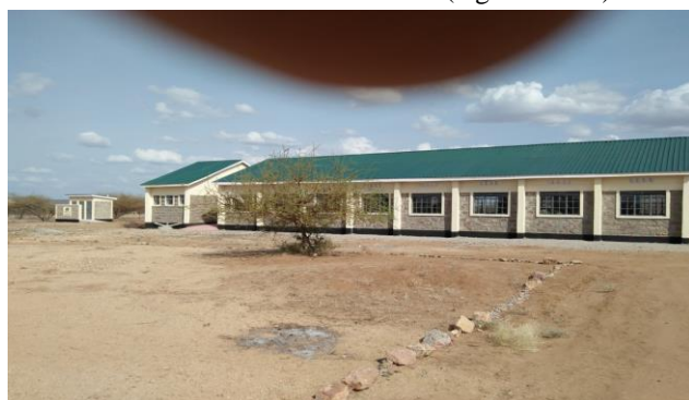
Photo 4.2 – Classrooms Block (Ngamia One)
