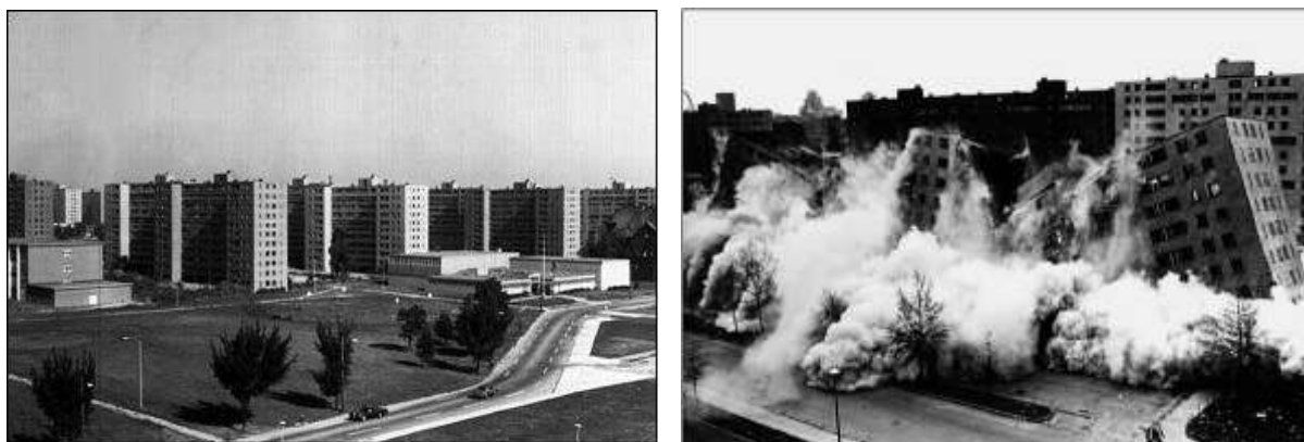
Fig. 2 – Before and After demolishing the Pruitt - Igoe
